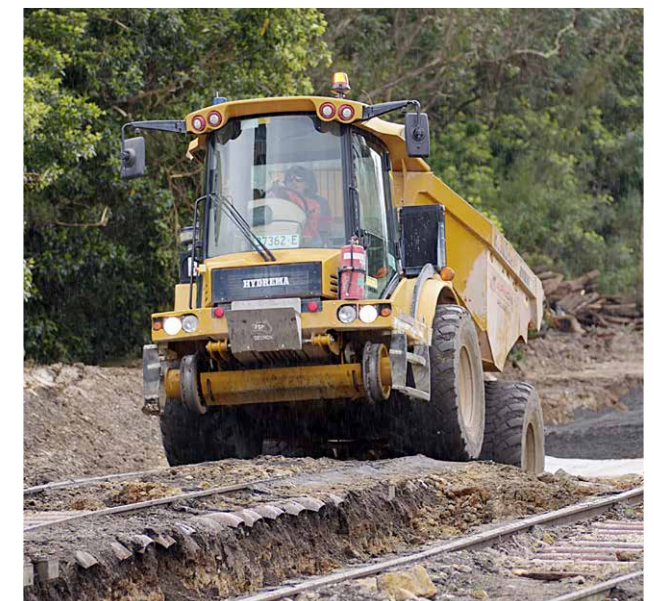
Track works underway at Colo Vale.
