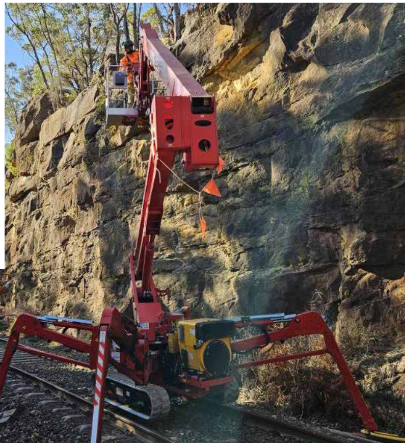
Geotechnical works kick off in cuttings along the Loop Line.
