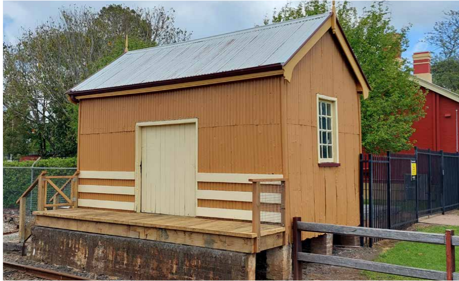
▼ The restored Goods Shed platform at the NSW Rail Museum.
