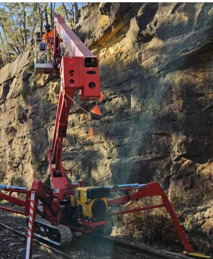
Geotechnical works kick off in cuttings along the Loop Line.
