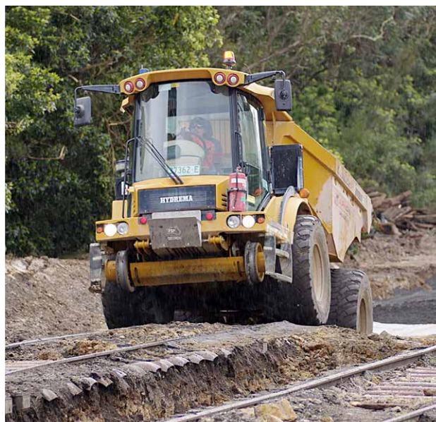
Track works underway at Colo Vale.
